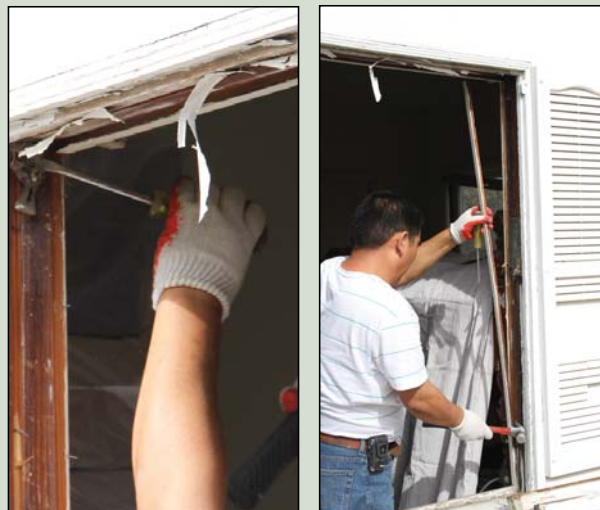
Remove old side trim, nails, and screws
