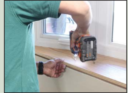
6. Drill Screws on Board
